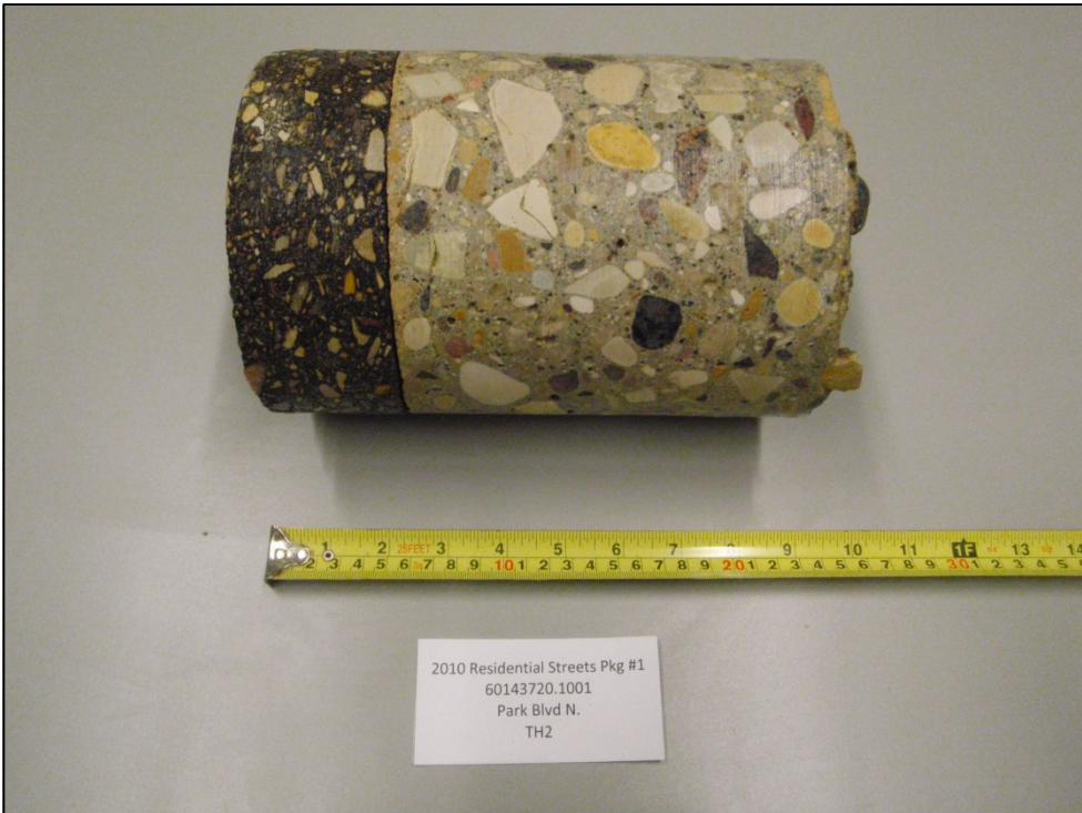
Photograph 2. Park Blvd N. – TH2
